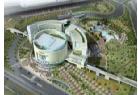
Gimpo Airport Sky Park Hot water / 700RT 13 units
