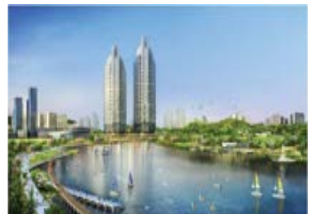
POSCO Gwanggyo Residential Complex Hot water / 525RT 3 units, 135RT 2 units
