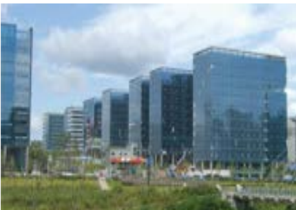
Pangyo Mtek Vision Office Hot water / 600RT 3 units, 340RT 10 units
