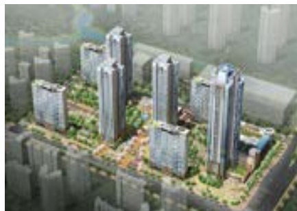
Lotte Cheongna Residential Complex Direct Fired / 500RT 2 units
