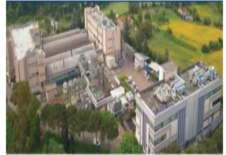
IBI Pharmaceutical Spa in Italy Hot water / 180RT 1 unit
