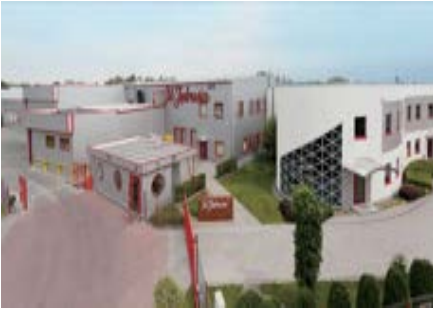
JEDRUS in Poland Hot water / 90RT 2 units
