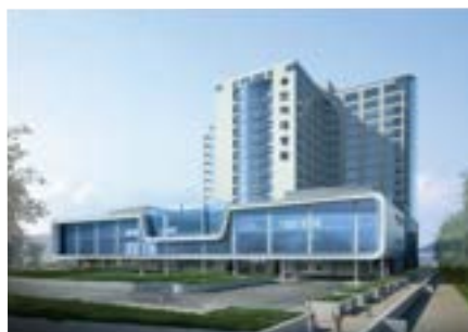
Inha University Hospital Direct Fired / 800RT 4 units
