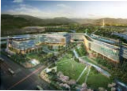
Government Complex in Sejong City Administrative Complex Hot water / 600RT 8 units
