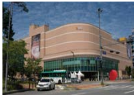
E-Mart (Paju Unjeong / Asan Baebang) Hot water / 575RT 2 units, 525RT 2 units
