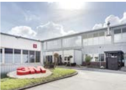
3M - Hilden in Germany Hot water / 240RT 1 unit
