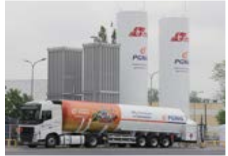
PGNiG in Poland Direct Fired / 180RT 1 unit
