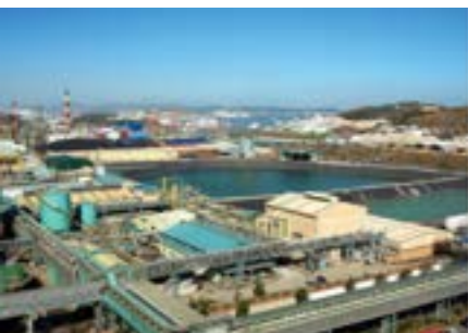
Korea Zinc Onsan Refinery Steam / 500RT 2 units
