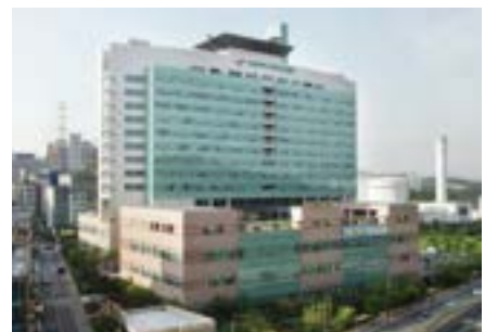
Dongtan Hallym University Hospital Hot water / 900RT 2 units
