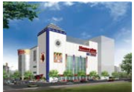
Homeplus Sosa Direct Fired / 600RT 5 units
