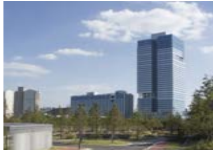
Heungdeok IT Valley Hot water / 825RT 2 units, 270RT 2 units, 155RT
