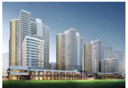
Lakeside Gwanggyo Residential Complex Hot water / 675RT 2 units, 525RT 2 units
