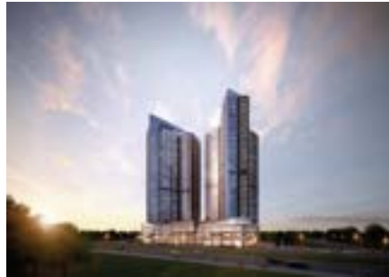
Songdo Landmark Prugio City Hot water / 600RT 2 units, 400RT units, 200RT units
