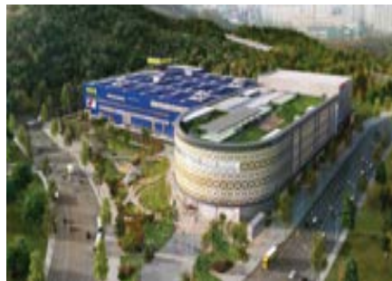
Gwangmyeong Lotte Outlet Hot water / 600RT 7 units, 135RT 2 units
