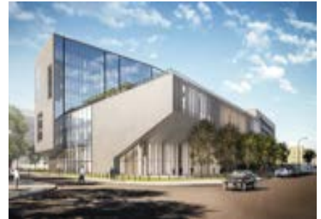
SYMBIOSIS MILANO in Italy Hot water / 75RT 1 unit
