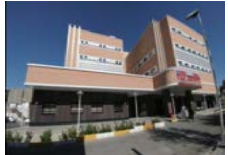
Bahar Hospital in Iran Steam Fired / 500RT 2 units
