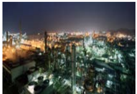
Lotte Chemical Yeosu Plant Hot water / 525RT 2 units, Steam 1100RT
