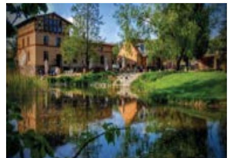
Tornow in Germany Hot water / 75RT 1 unit
