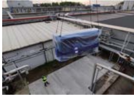
Hospital Trigen in Poland Hot water / 60RT 2 units
