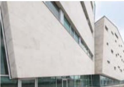
Tehran Hospital in Iran Direct Fired / 360RT 1 unit
