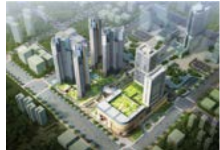
Lotte Department Store Dongtan Hot water / 820RT 10 units, 280RT 2 units
