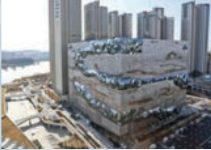
Galleria Department Store Gwanggyo Hot water / 750RT 6 units, 190RT 2 units
