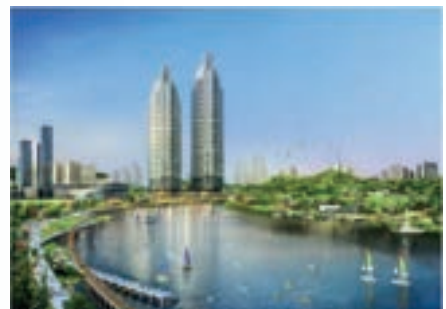
POSCO Gwanggyo Residential Complex Hot water / 525RT 3 units, 135RT 2 units
