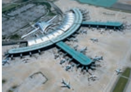
Incheon International Airport Hot water / 975RT 8 units
