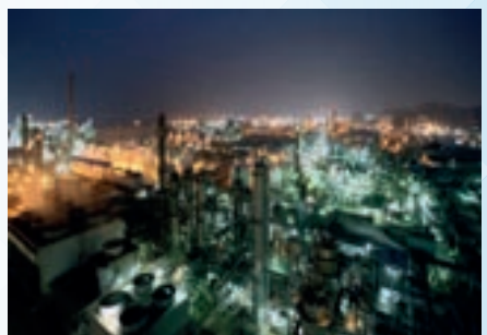
Lotte Chemical Yeosu Plant Hot water / 525RT 2 units, Steam 1100RT
