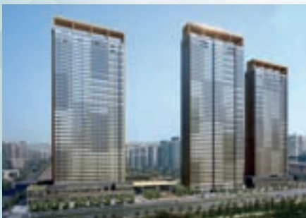
Lotte Songdo Residential Complex Hot water / 470RT 2 units, 340RT 4 units
