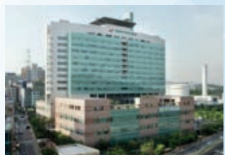
Dongtan Hallym University Hospital Hot water / 900RT 2 units
