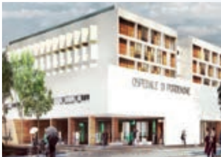
Pordenone Hospital in Italy Hot water / 210RT 2 units
