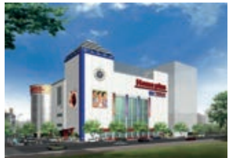
Homeplus Sosa Direct Fired / 600RT 5 units
