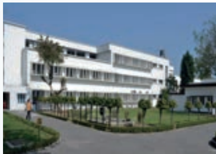
R&D Center in Iran Direct Fired / 240RT 1 unit
