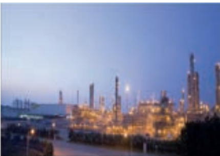
Lotte Chemical Daesan Plant Hot water / 1,300RT 3 units, 975RT 1 unit
