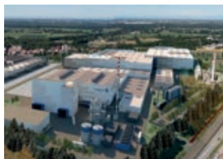
Vetropack in Italy Hot water / 155RT 2 units
