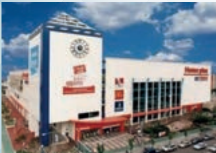
Homeplus Suwon Homesil Hot water / 600RT 2 units
