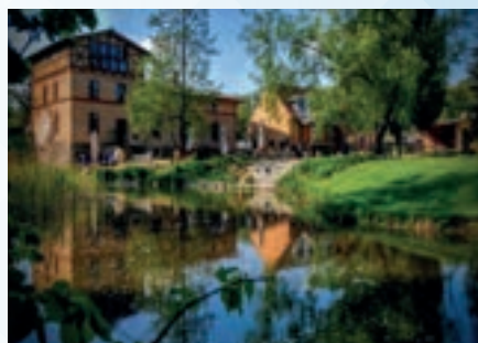
Tornow in Germany Hot water / 75RT 1 unit
