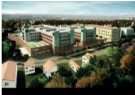
New Treviso Hospital in Italy Hot water / 420RT 1 unit
