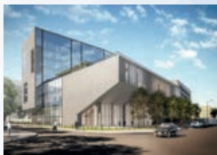
SYMBIOSIS MILANO in Italy Hot water / 75RT 1 unit
