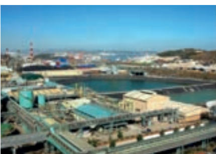
Korea Zinc Onsan Refinery Steam / 500RT 2 units
