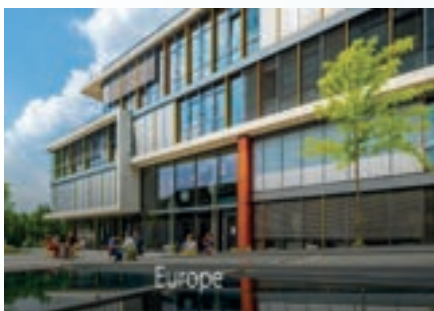
Militeny Biotec in Germany Hot water / 90RT 2 units
