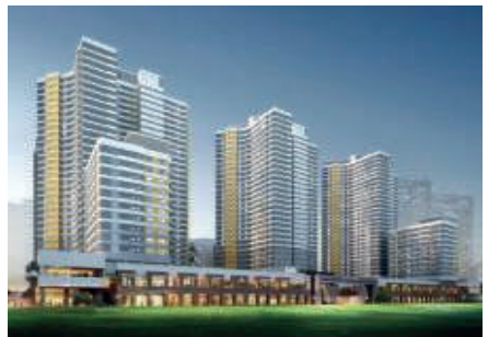
Lakeside Gwanggyo Residential Complex Hot water / 675RT 2 units, 525RT 2 units
