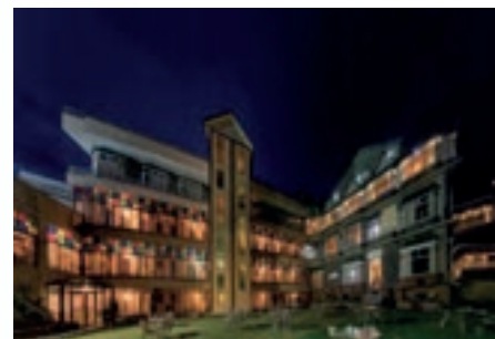
Hotel OA in Pakistan Hot water / 240RT 1 unit
