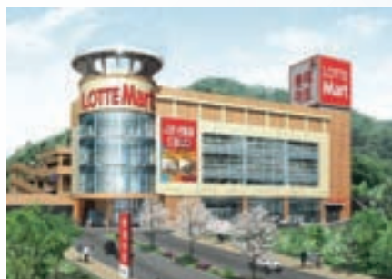
Lotte Mart Suwon Branch Direct Fired / 700RT 6 units
