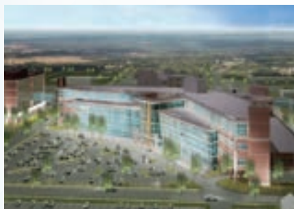
Karachi Hospital in Pakistan Hot water / 375RT 1 unit
