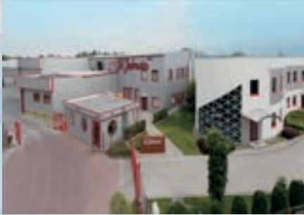
JEDRUS in Poland Hot water / 90RT 2 units
